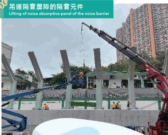
安裝和固定隔音屏障的鋼柱 Installation of steel post of the noise barrier
