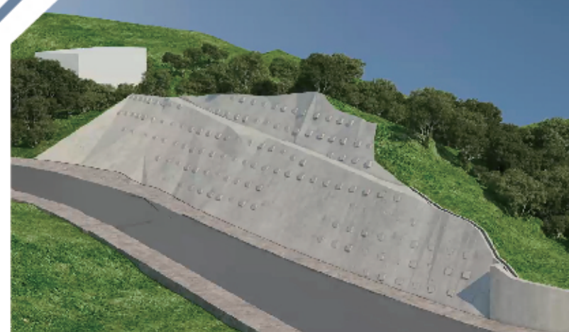
青榕街斜坡及護土牆優化設計 Revised Design of Slope Works and Retaining Wall at Tsing Yung Street
